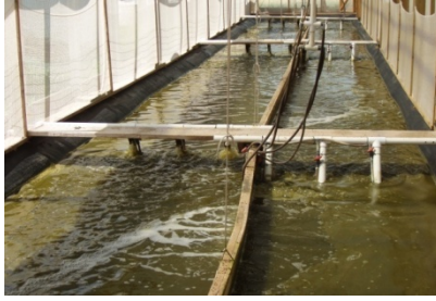
Figure 1: A general view of a raceway full of water
